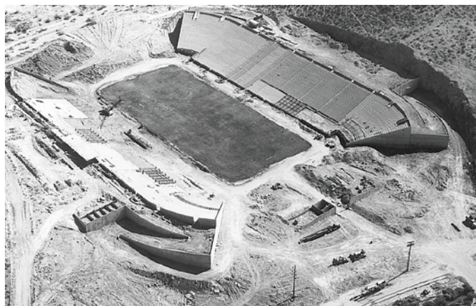
Sun Devil Stadium construction in progress in 1958.
